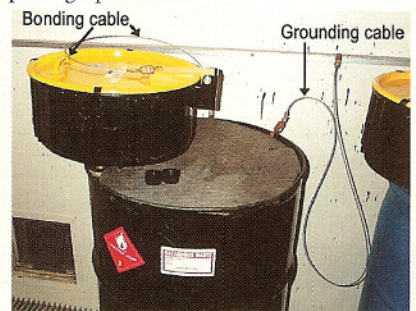
This photo illustrates flammable solvent being placed inside a 55-gallon waste drum. The funnel is bonded to the drum and drum is grounded. Source: Author's collection.
